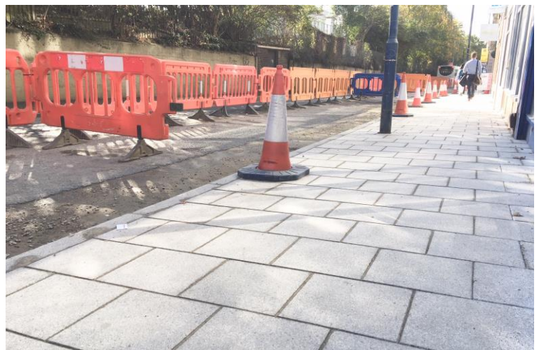
High Street new paving stones
