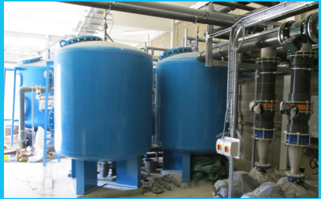
The water pumps and filters for both pools have been installed.
