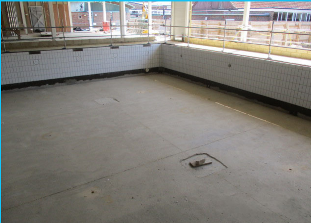
Teaching pool being tiled ahead of the moveable floor being installed at the end of July.
