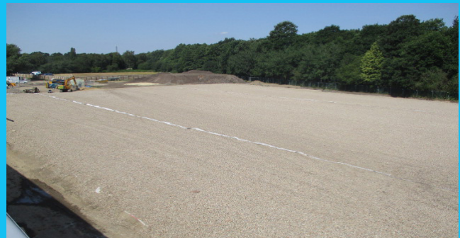
The surface of 3G pitch has been prepared. During July the edging will be installed, followed by layers of stone and tarmac, which make up the underside of the playing surface.
