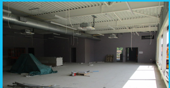
Main fitness area on the first floor being fitted out.
