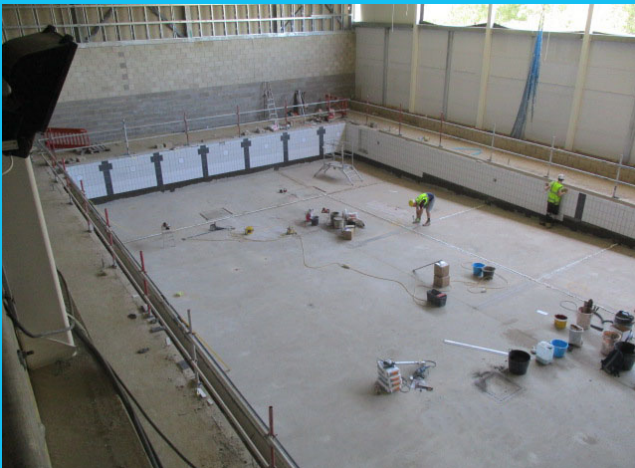
Tiling of the main pool will be completed by mid July.
