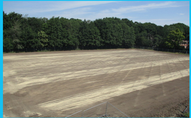
The rugby pitch has been completed and seeded.
