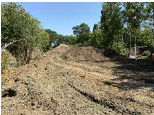
7,000 cubic metres of material was screened on site
