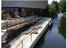
Works have been going on to construct a brand new pedestrian and cycle bridge, uniting the two sides of the canal path, and the reflection of the gabion walls and polished steel railings on the water show a project excitingly close to completion. Just the connecting section remains to be built.
